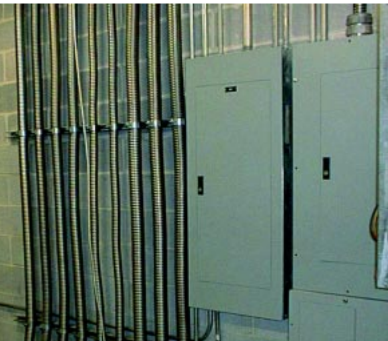
Photo 9. Supporting MC cable every six feet.
