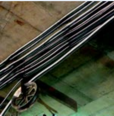
Photo 2. MC cable pulled over sheave wheel
