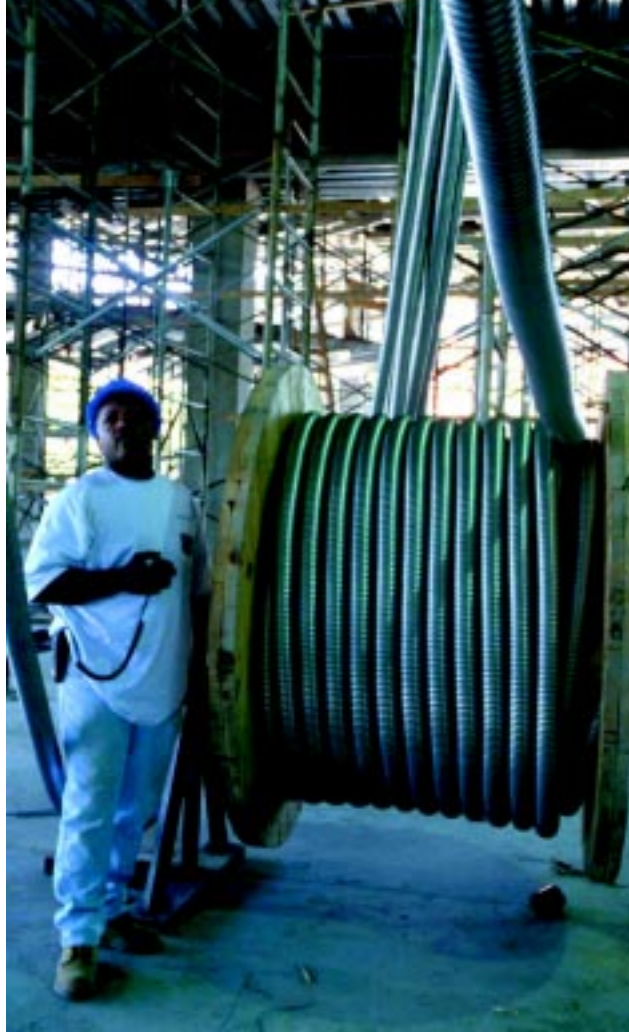
Photo 10. Paying off large size MC cable.
